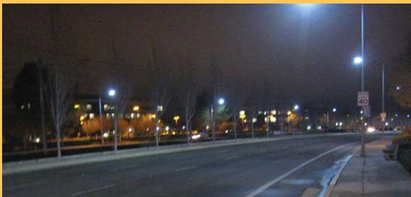
LED Streetlight Project
